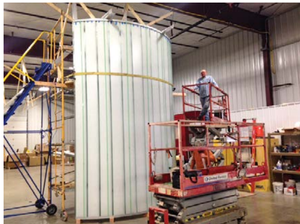
Prefabrication of the channel glass in a controlled environment led to quicker installation.
