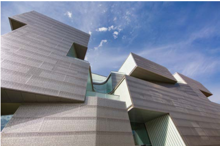
During the day, the façade of the Visual Arts Building at the University of Iowa acts as a sunshade to the hidden windows behind it. This design also provides a light, porous aesthetic touch.
