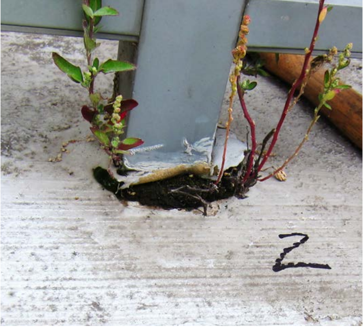
Weathered grout with biological growth.
