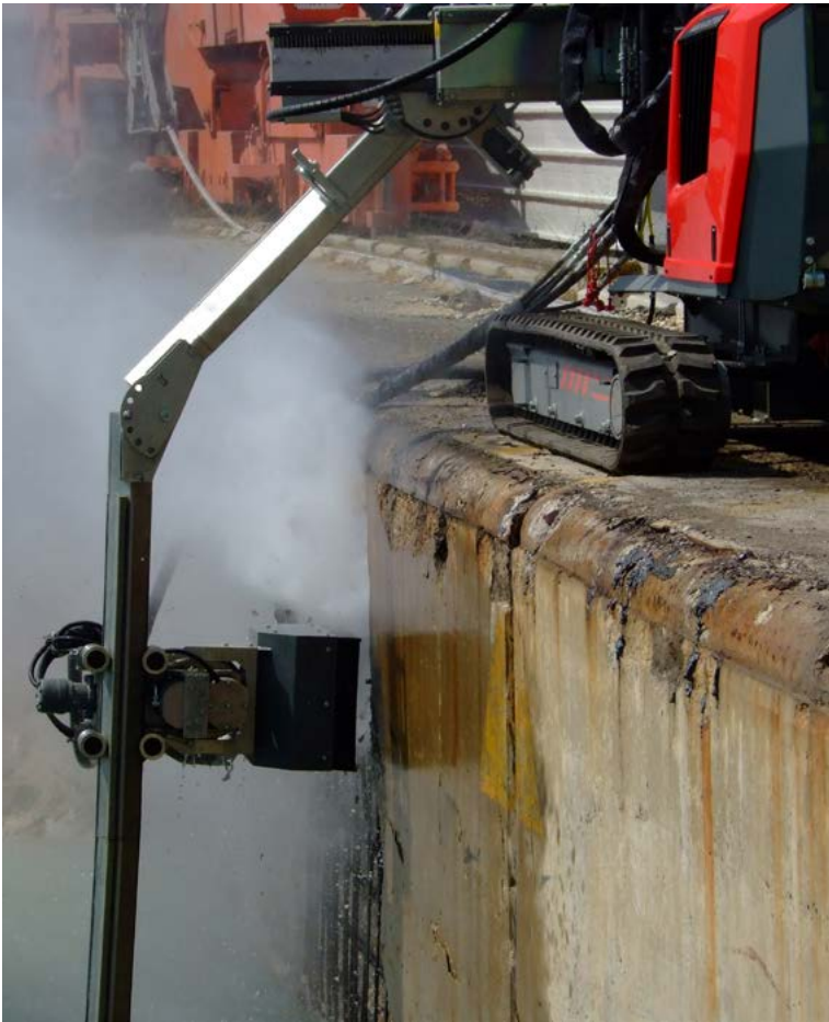
Hydro-demolition can remove old concrete while doing repair work without creating micro-fracturing and the future need for additional patch and repair materials.
