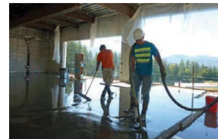
SUPERCAP® is proactively placed after the base slab was bull floated in Division 3
