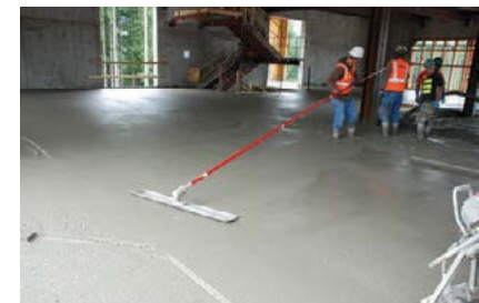
The slab is bull floated
