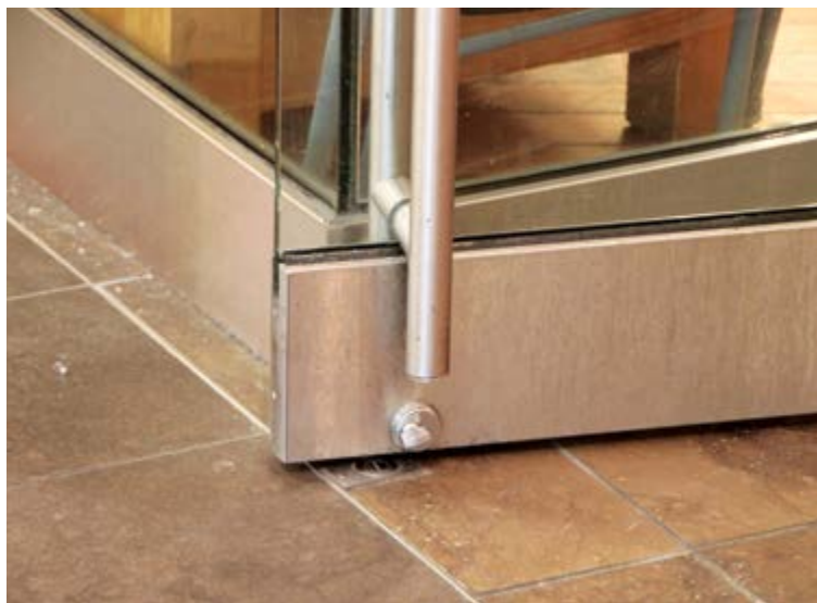
Manual doors on an accessible route must have a smooth surface on the push side with no protruding hardware within 254 mm (10 in.) of the floor or ground. In the photo above, these components could inhibit passage through a door opening by catching a crutch, cane, walker, or wheelchair.
