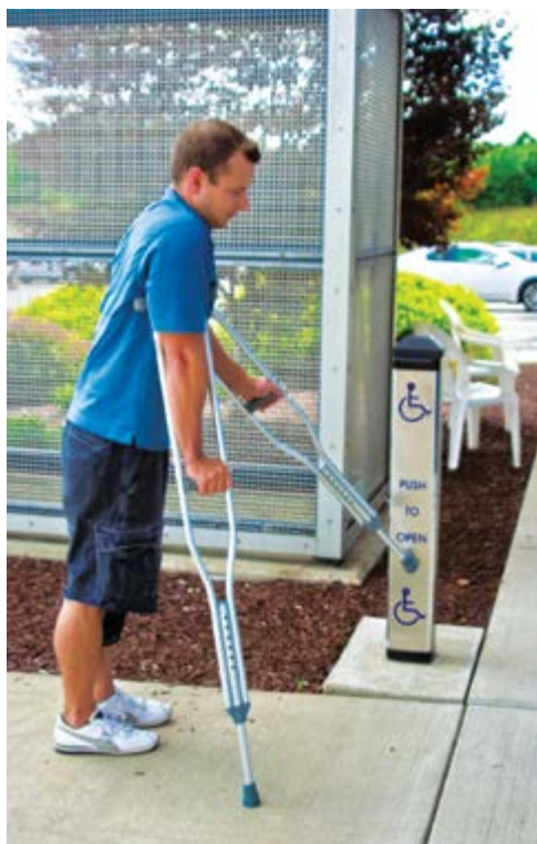
Some jurisdictions require actuators mounted in two positions, or a vertical bar actuator that will allow the door to be operated by a hand/arm or a crutch, cane, or wheelchair footrest.
