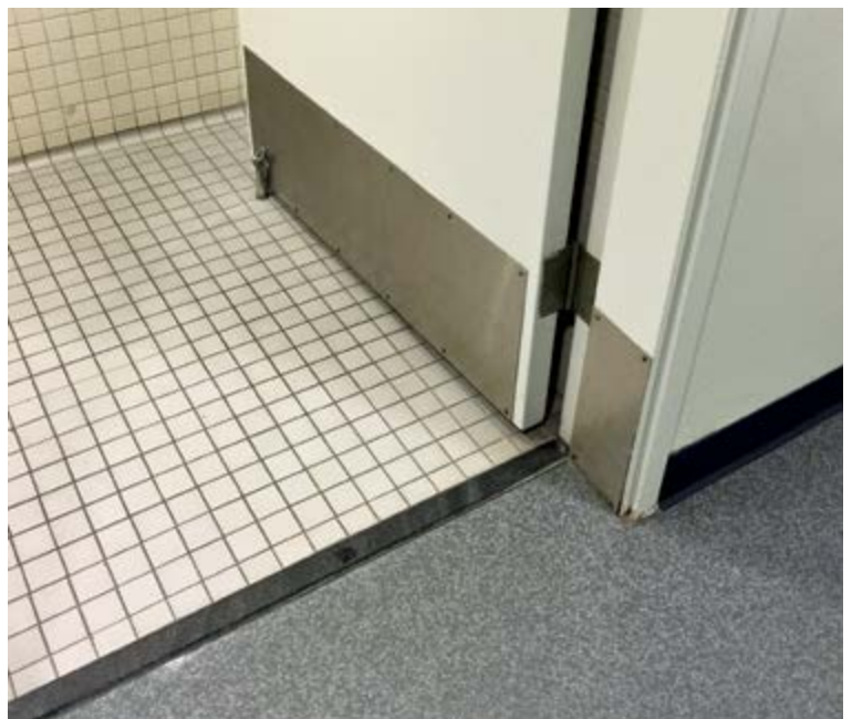
A kickplate, also known as a protection plate depending on its height and application, is used to protect the face of the door in high use and abuse areas. This way, the face of the plate withstands the damage or elements, and can be replaced at a lesser cost than the replacing the door. Although available in most finishes, stainless steel is the most common.
