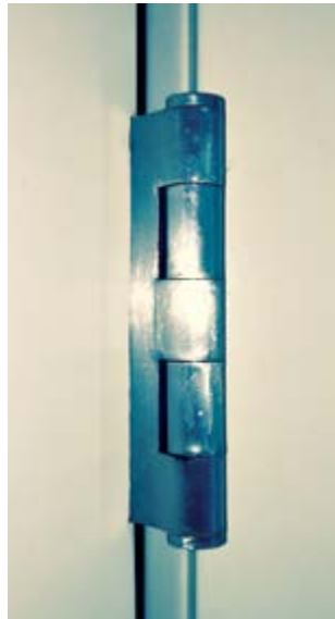
A five-knuckle non-bearing hinge is one of the most commonly used hanging devices, along with the bearing five-knuckle hinge. Non-bearing hinges allow the knuckles to rub together, causing wear of the metal over time, while bearing hinges allow for a smoother operation and less friction.
