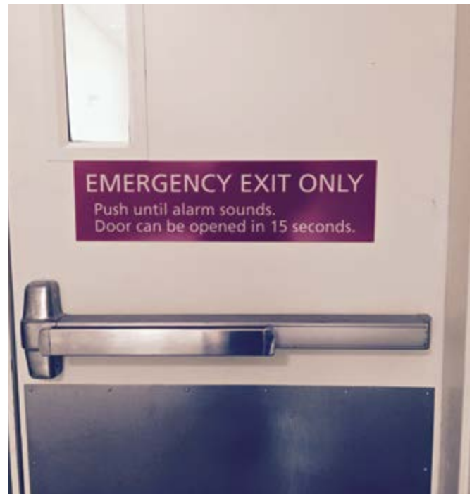
Delayed egress fire exit hardware delays the release of the latch from the egress side with the intent to allow time for a responder, while not keeping the person in danger for longer than necessary.
