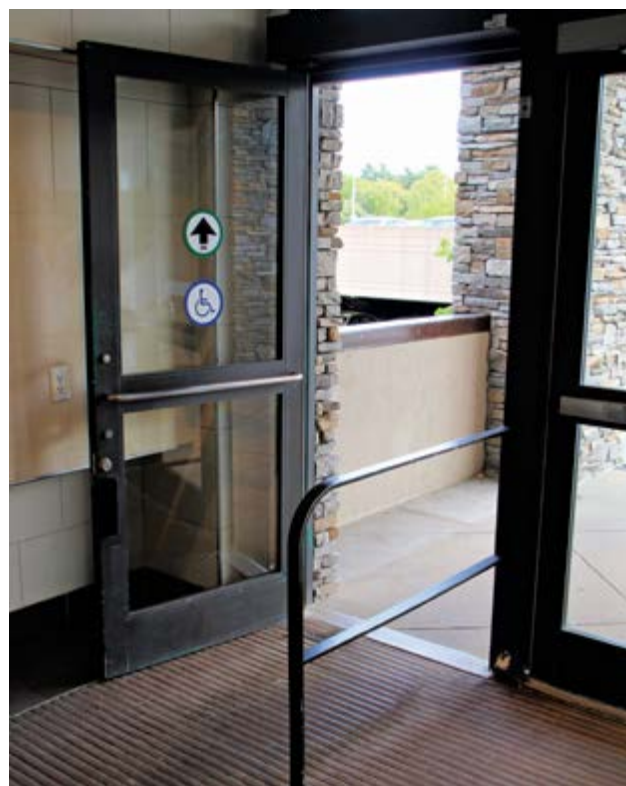
If a motion sensor is used to actuate a door with an automatic operator, then guide rails and safety sensors are typically required.
