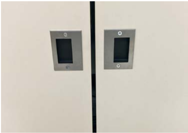
Flush pulls are an option for doors that do not require a locking or latching device—a publicly accessible closet might be an ideal application. Other reasons to choose pulls over locks or latches could be for the design intent or cost.
