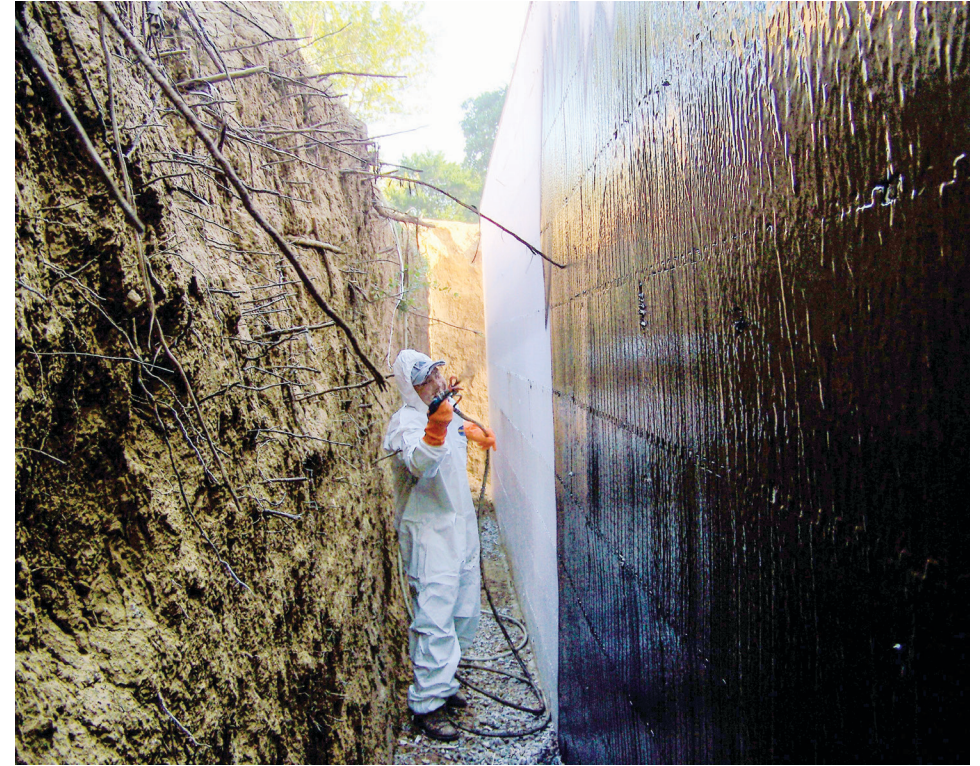
Spray installation of polymerized asphaltic emulsion.
