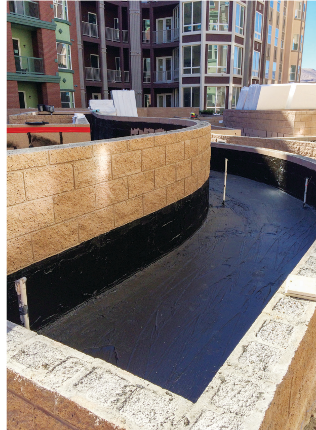
Finished planter box installation of polyether membrane.
