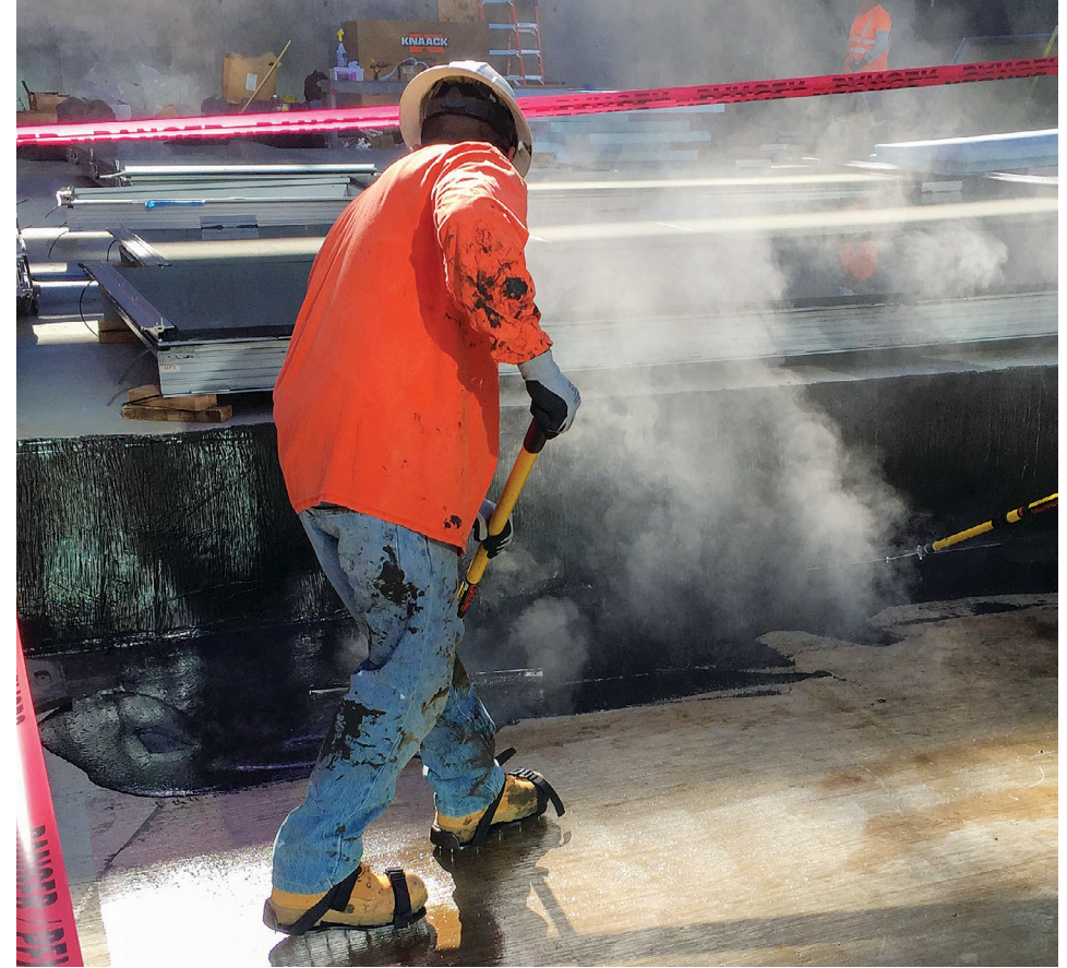
Installation of hot rubberized asphalt membrane.
