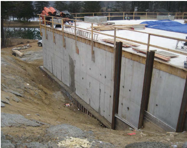
This image shows initial leaks in concrete during the construction of a new facility at the Newburyport Wastewater Treatment Facility (NWWTF) in Massachusetts.
