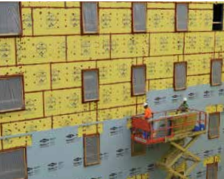
The DensElement® Barrier System installed on Eagle's Landing Apartments, Burlington, Vermont.
