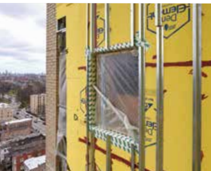
DensElement® Barrier System integrated into wall assembly, Fannie Emanuel, Chicago, Illinois.
