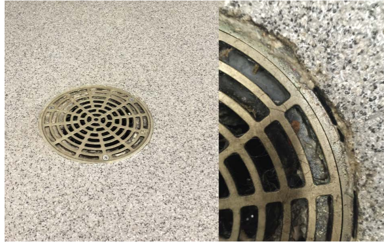
Examples of both good and bad drain terminations shows chipping and delamination at the drain.
