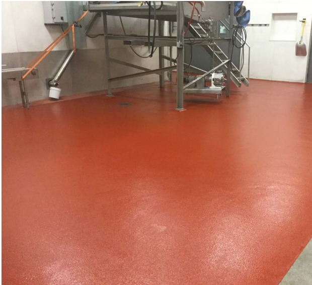
Urethane cement used in food processing area.
