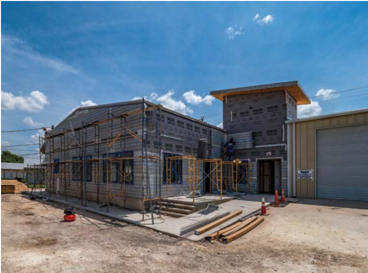
The exterior of the fire station is made up of stucco cladding. This design required a durable building envelope that could withstand the notoriously hot and humid climate in Texas with a focus on airtightness and vapor permeability.
