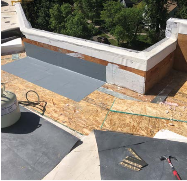
Roof vapor/air barrier at roof perimeter.
