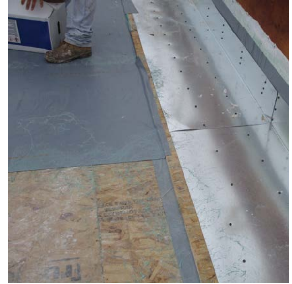
Vapor/air barrier applied to field of roof.
