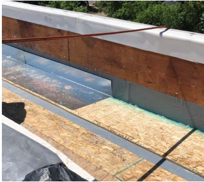
Plywood and sheet metal angle parapet reinforcement.
