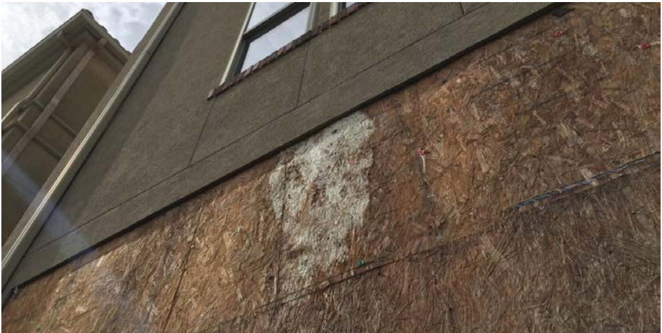
Moisture damage on wood-frame, low-rise building.
