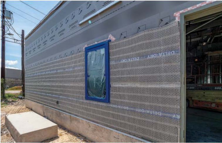
Ventilated rainscreen membrane that is made of a special high-density polyethylene (HDPE) with pre-installed glass lath.
