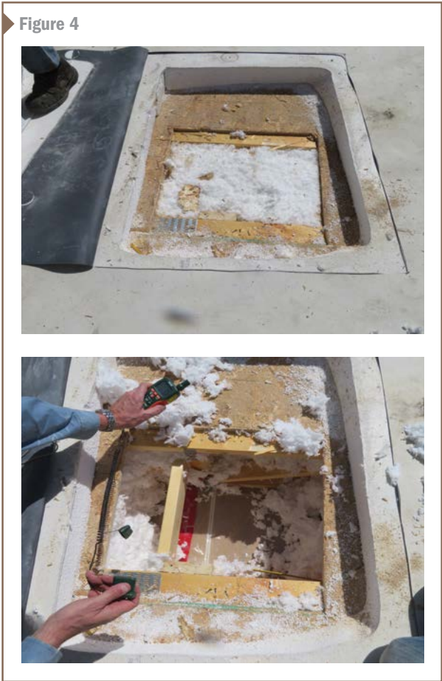
Typical invasive inspection opening above trusses (top) and below roof deck sheathing (bottom).
