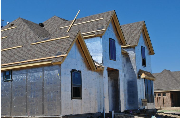
A wall with polyiso ci can achieve the code-required, minimum R-value with thinner materials than other products. Photo courtesy Rmax
