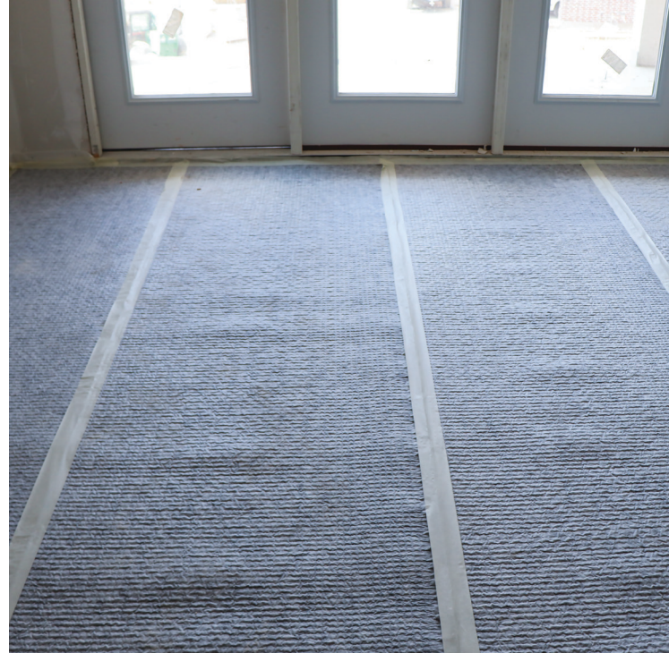
Properly installed sound mat covered with a layer of gypsum underlayment provides long-term benefits for property owners and residents.
